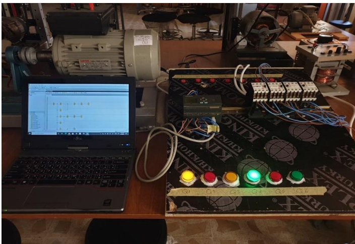
Fig. 2 Connection of PLC with induction motor
